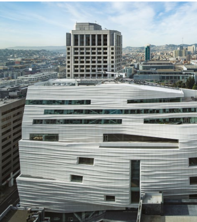
Inspired by the water and fog of San Francisco Bay, the expanded SFMOMA’s façade showcases the architectural possibilities of FRP.
